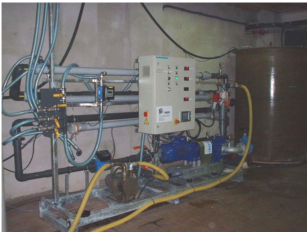
Figure 1.4: Membrane pilot-plant for degreasing liquor recovery
