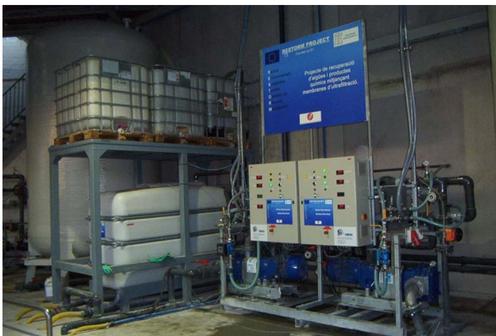
Figure 1.3: Membrane pilot-plant for lime liquor recovery
