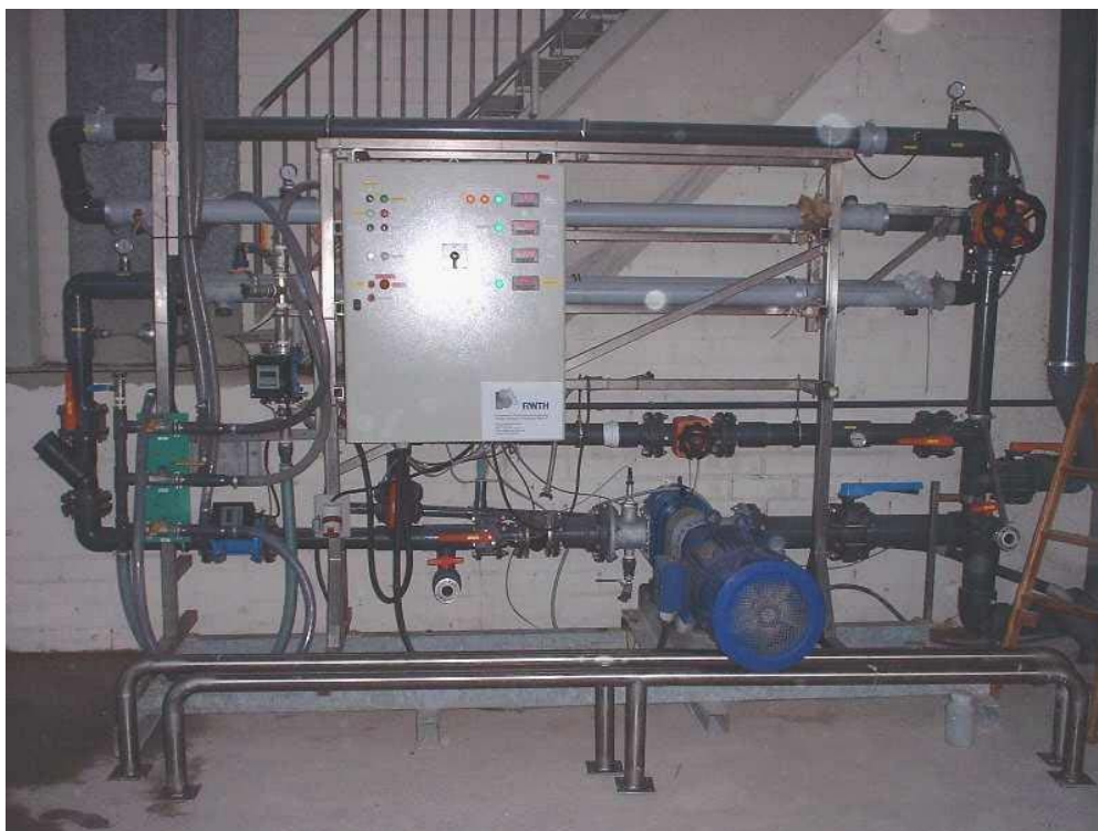
Figure 1.2: Membrane pilot-plant for soak liquor recovery
