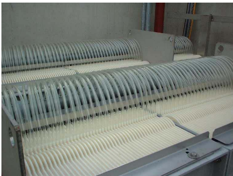
Figure 1.6. Submerged plate membranes in a Membrane Bioreactor
