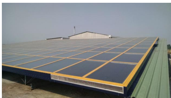
Fig. 13. A view of solar hot air collectors
