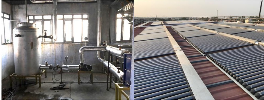
Fig 9 & 10: Solar water heating system
