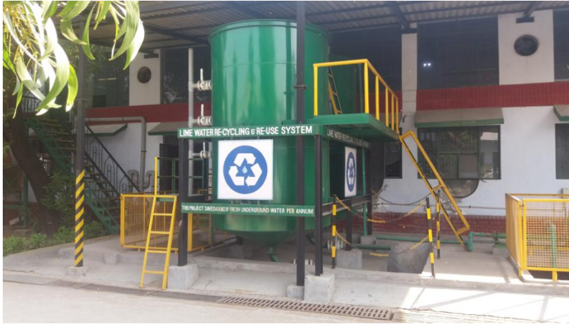
Fig. 19: A view of lime liquor recycling system
