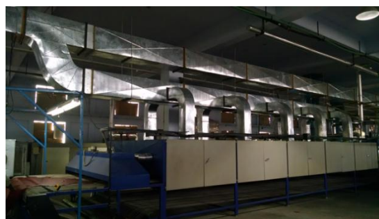
Fig.14: Ducting arrangement to introduce hot air in autospray drier
