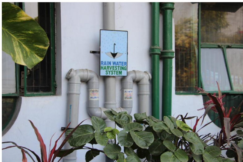
Fig 20: Pipeline and filter arrangement in rainwater harvesting in Kings International
