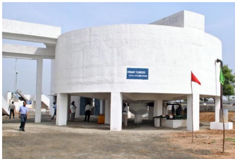
Elevated Primary clarifier
