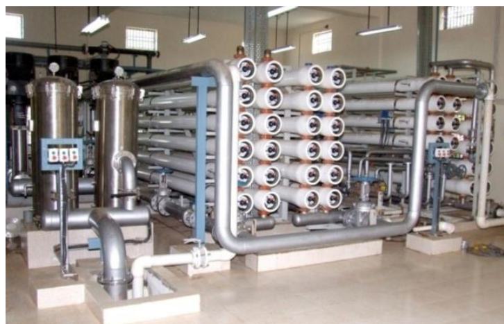
Fig. 3 - Reverse Osmosis system following MBR / UF
