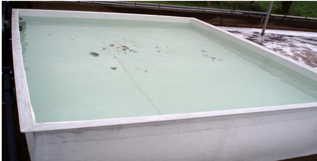
Picture: 2: Holding Tank with Nanofiltration permeate for water recycling
