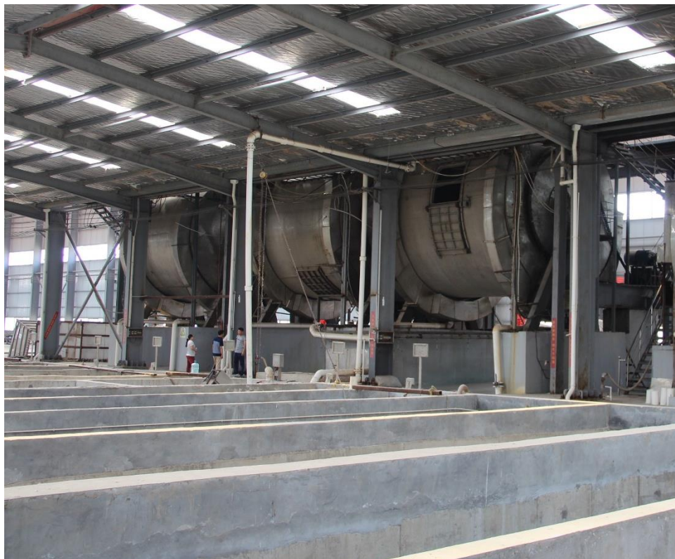
Figure 1 The BIOSK development plant
