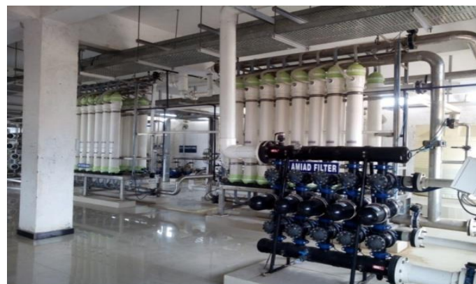
Fig. 2 - Amiad Filter & Ultra-filter (UF)
