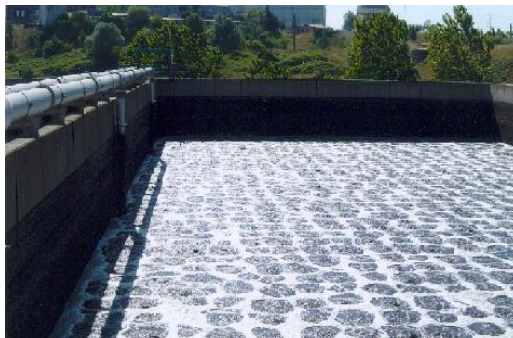
Fig. 10 - CETP in Istanbul, Turkey with Sea discharge for TDS management
