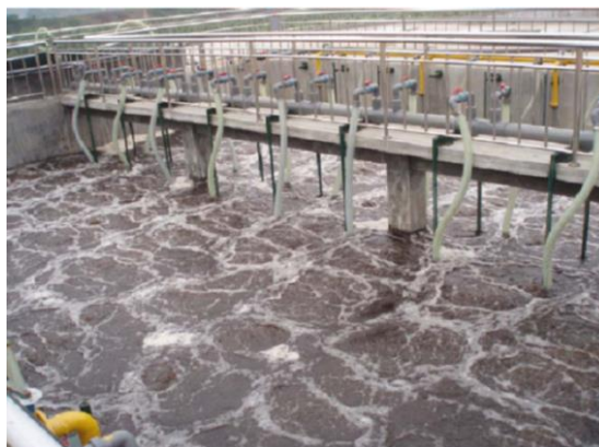
Fig. 4 - Submerged Membrane Bioreactor
