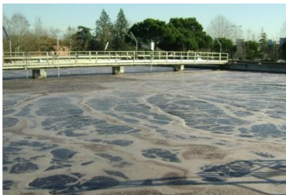
Fig. 6 – Extended Aerobic oxidation for sludge reduction in a CETP, Italy
